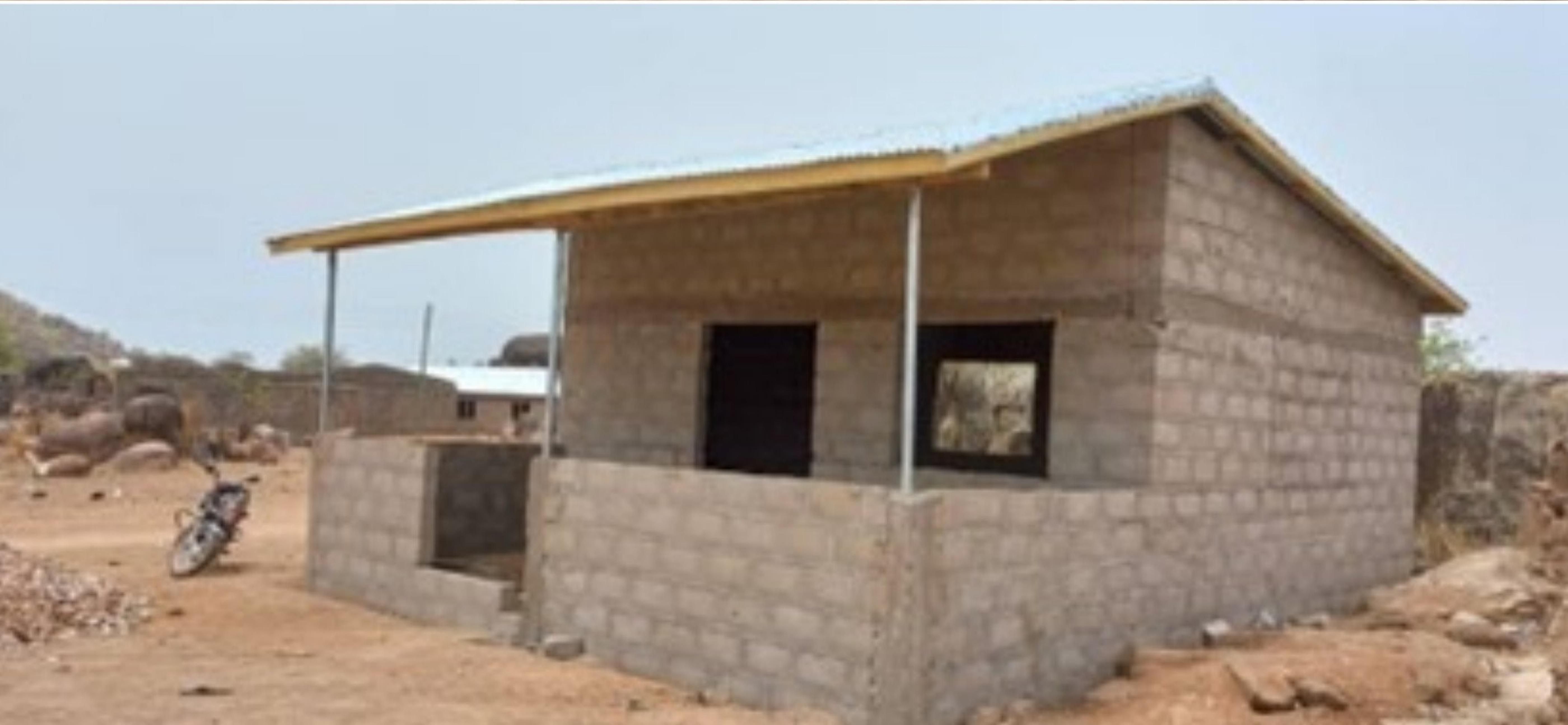
Picture 3: Wakii Rice process under construction
