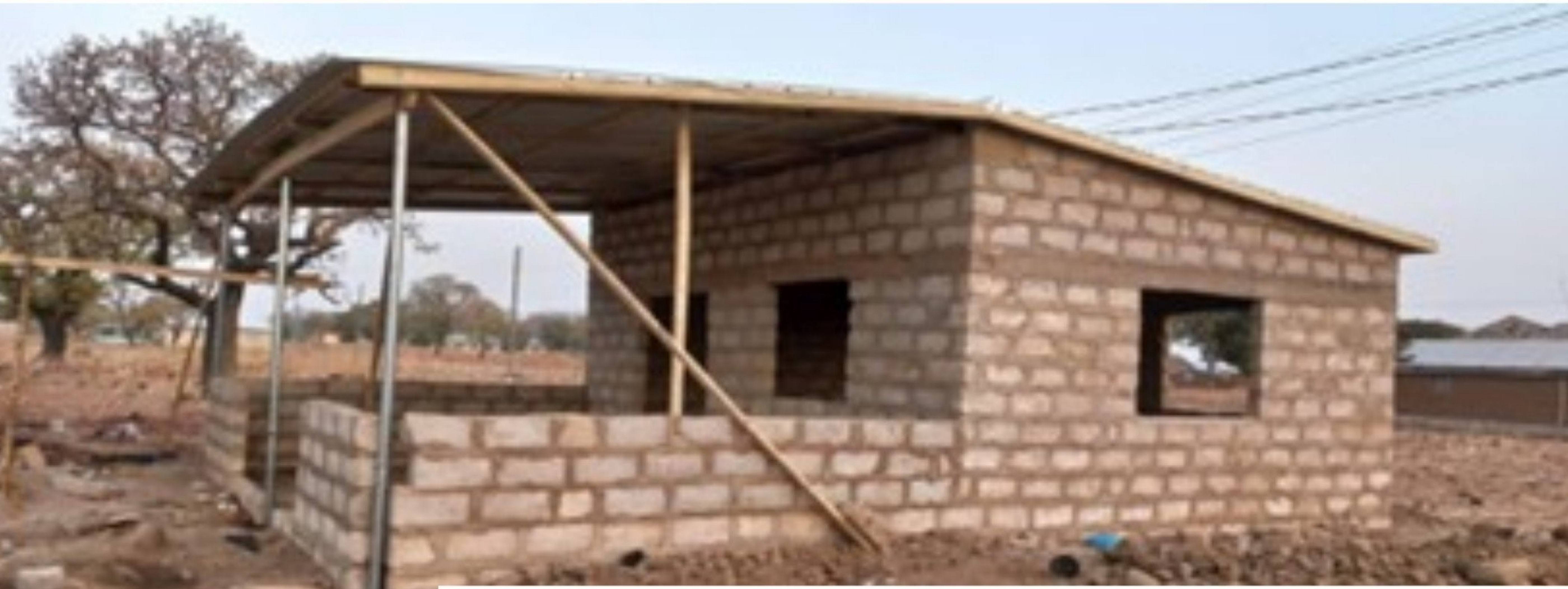
Picture 2: Anateem shea butter processing centre under construction
